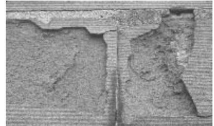
removal of all deteriorated stone down to solid material. The sound stone is then scarified or roughened to provide some mechanical anchorage for the composite patch. For large repairs, rods and wire armatures are sometimes added to provide additional support and to assure that the patch does not separate from the substrate. The rods can be made of fiberglass, nylon, or stainless steel. A durable composite repair must be at least 3/4” thick.
