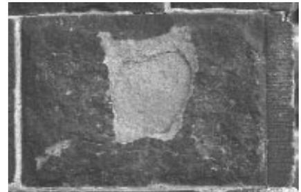
*Contour scaling (top) and disaggregation (bottom) are two commonly found forms of brownstone deterioration.*
