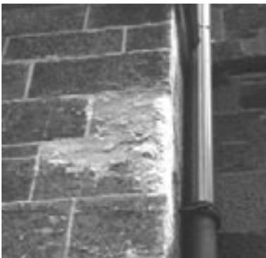
*Inappropriate repair methods, such as painting (top) and cementitious coatings (bottom), tend to trap moisture and mask underlying brownstone deterioration.*
